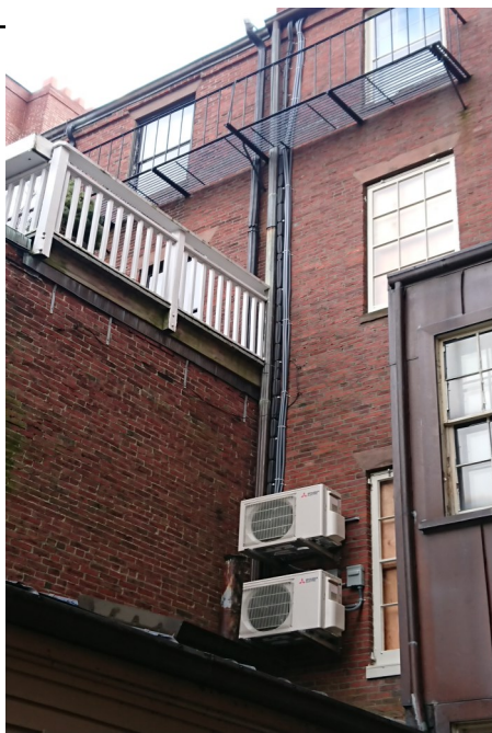
Air-cooled condensing units for 4th floor.
