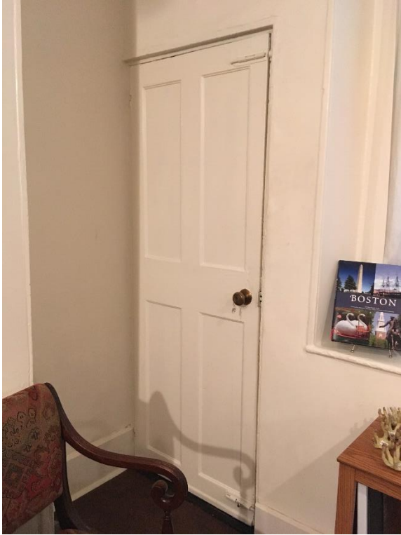
Figure 2: Door to the closet stack/staircase on first floor. This door is in the kitchen which is currently used as a greeting space and gift shop.
