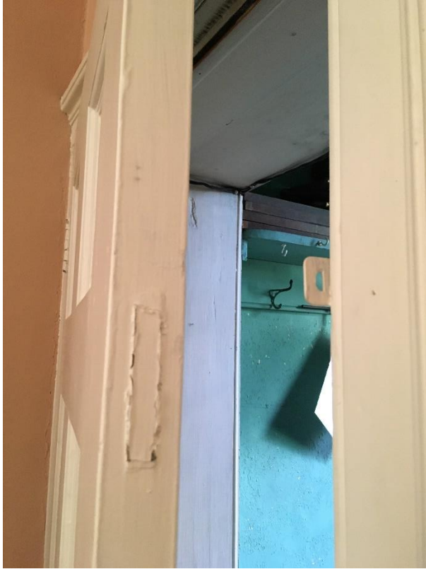
Figure 14: The door and frame for the third floor bedroom closet shows the presence of hardware that has been removed. There is no longer a rod or beam at the top of the door to slide through the metal slot on the right, but this suggests that there was once another way to bolt the door shut from within the bedroom, blocking access for any entering from, perhaps, an external stair.
