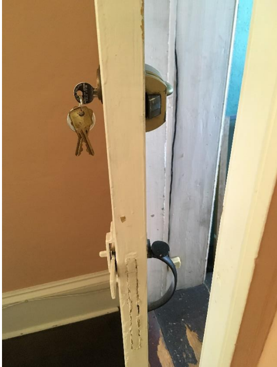
Figure 12: The door to the closet stack in the third floor bedroom shows the most layered use of hardware. In this image you see the original hardware on the bottom and the later key lock above, possibly installed by or for Mary King, though this is not a recorded date.
