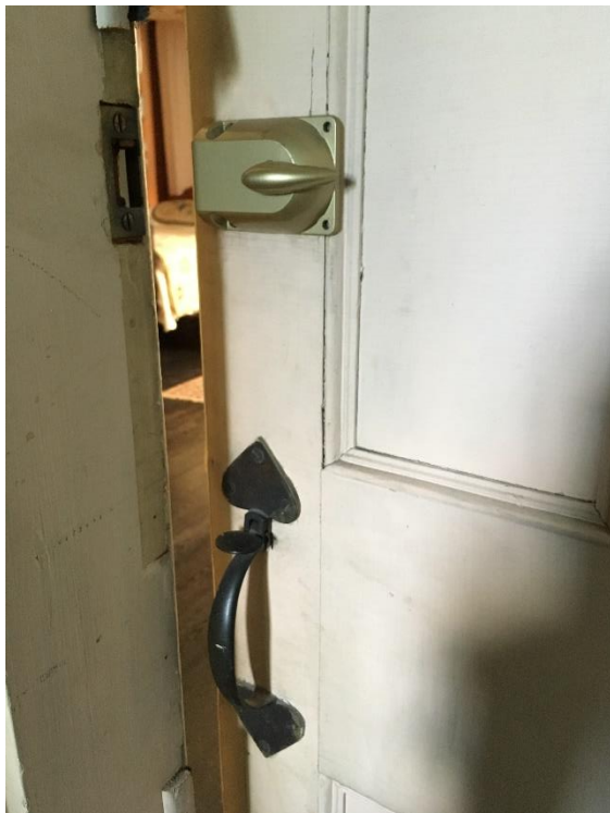
Figure 13: The hardware for the third floor closet, as viewed from inside of the closet itself. As seen here, there is a thumb latch for use when entering the room from within the closet.
