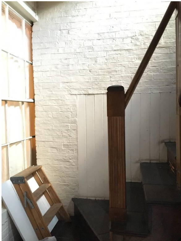
Figure 11: The first floor enclosure below the butler's pantry, looking onto the "closet stack."
